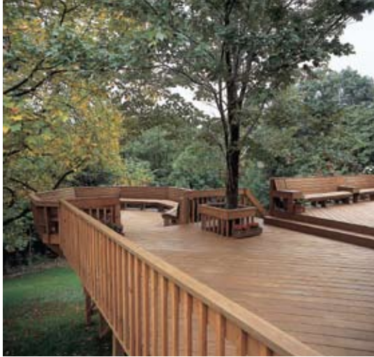
Deck coated with Wolman RainCoat tinted cedar.
