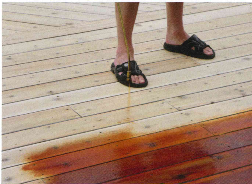
● Spraying the deck.
