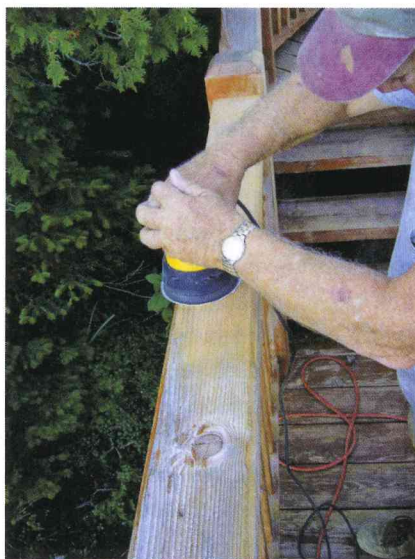
● Sanding the deck
