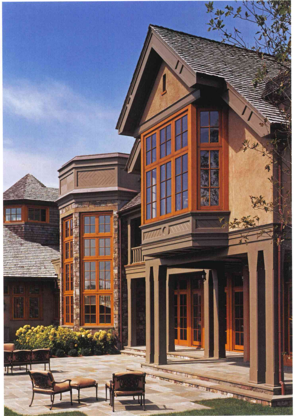
This home in upstate New York used a custom blended stain, top coated with the Hydrocrom clear water-based system from Italy's Milesi spa. Hydrocrom is exclusively imported by Colorspec Coatings International, Inc., Holbrook, NY. It is an elastomeric coating which means it remains flexible while maintaining lasting durability. Photo courtesy of Reilly Windows & Doors.
