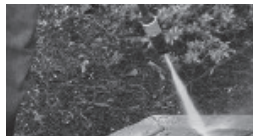
POWER WASH ENTIRE SURFACE
