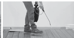
APPLY SANSIN SDF EVENLY BY BRUSH OR SPRAY APPLICATION
