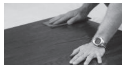
SAND TO REMOVE GLAZE AND IMPROVE ADHESION
