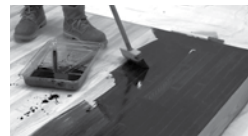
APPLY WITH A GOOD QUALITY BRUSH OR PAD APPLICATOR OR BY SPRAYING
