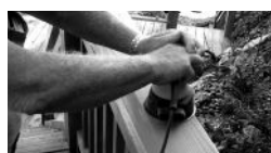
IF NECESSARY, FINISH SANDING
